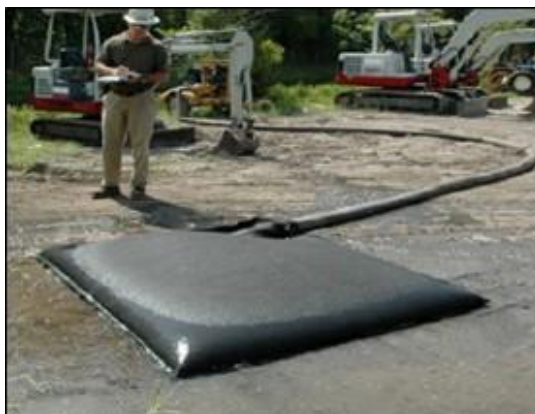
Plate 4-7 Silt Bag under inspection
