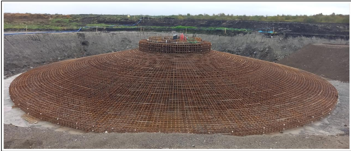
Plate 4-2 Turbine Base Anchor Cage surrounded by reinforcing steel.
