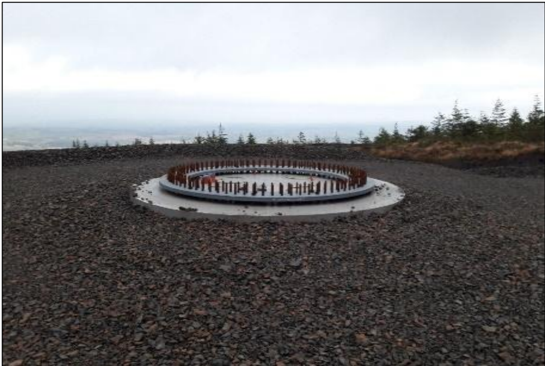
Plate 4-3 Finished Turbine Base
