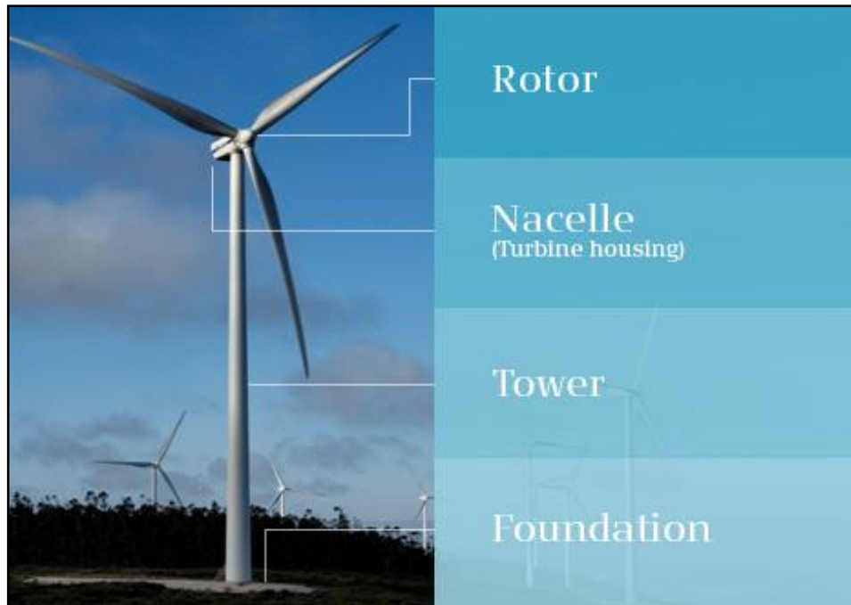
Plate 4-1 Wind turbine components
