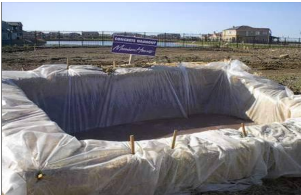
Plate 4-5 Concrete washout area
