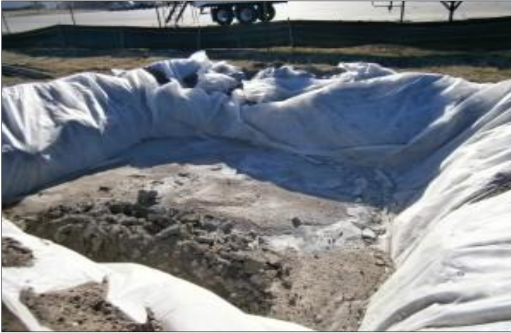
Plate 4-6 Concrete Wash Out Area
