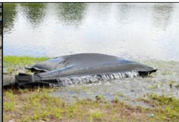
Plate 4-8 Silt Bag with water being pumped through
